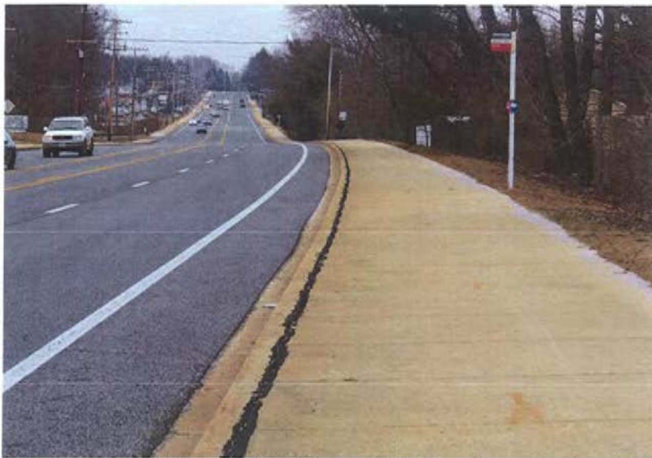
This wide outside curb lane along MD 197 was provided through narrowing the existing travel lanes. It provides additional space next to the curb to accommodate bicyclists, while also providing a striped buffer for pedestrians along the sidewalk.
