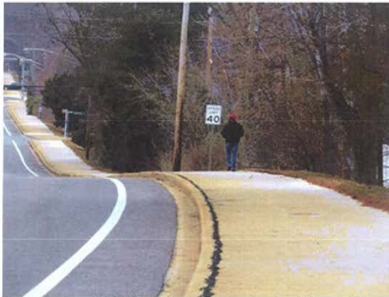
Restriping along MD 197 included narrowing the travel lanes and center turn lane to provide a wide outside curb lane to accommodate bicyclists and buffer the sidewalk.
