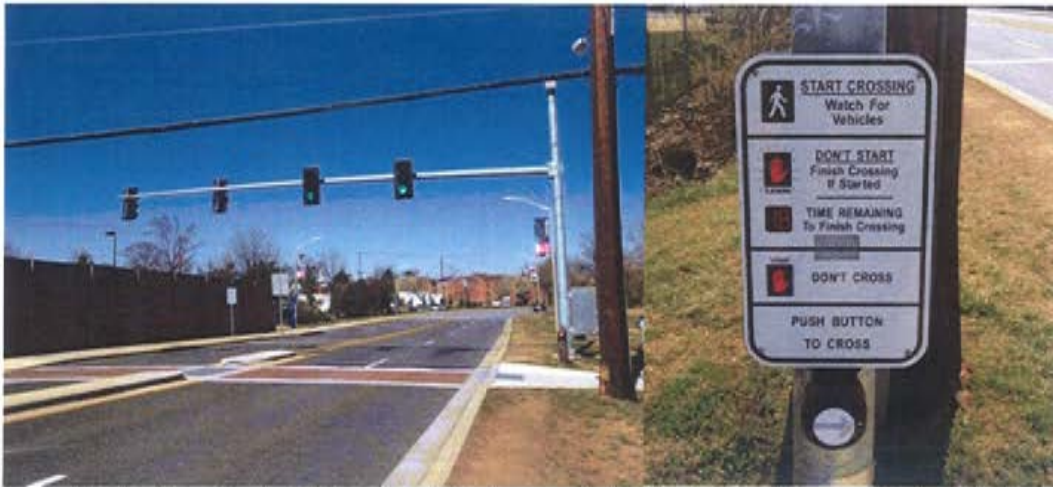
Full pedestrian signal at Paint Branch Parkway and the Rhode Island Avenue Trolley Trail.
