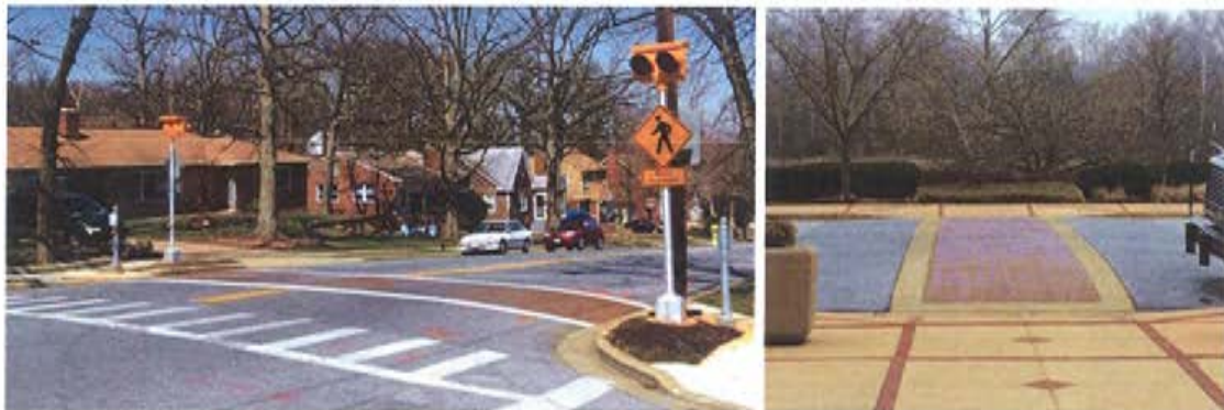
Raised crosswalk with hazard beacon on Cheverly Avenue (above left), Governor Oden Bowie Drive (above right)
