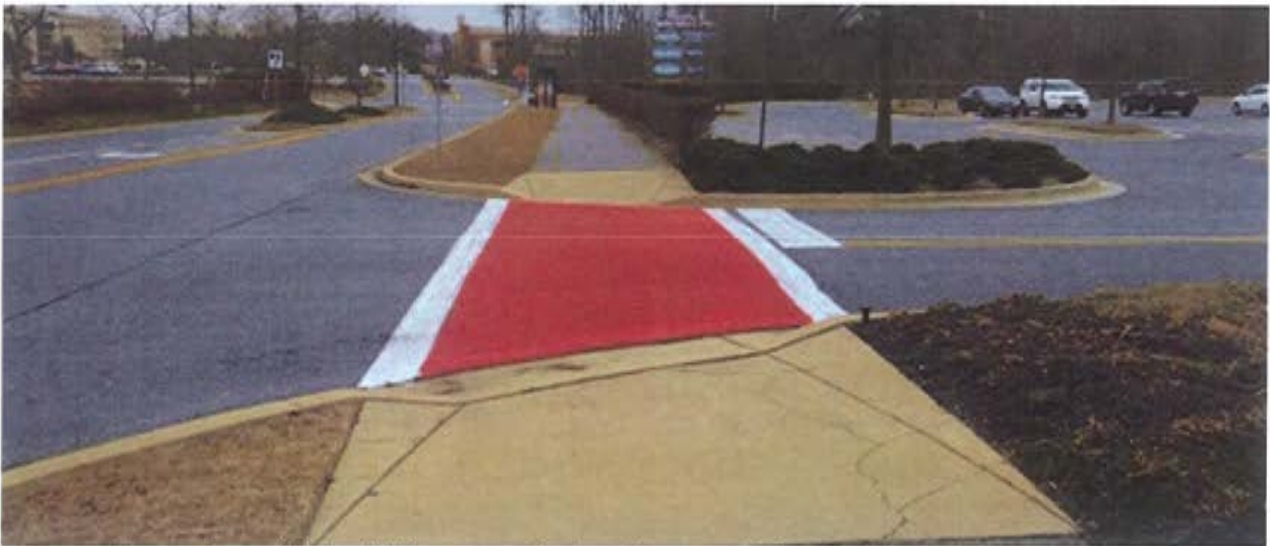
Contrasting and high visibility crosswalk along Evergreen Parkway at the Bowie Town Center
