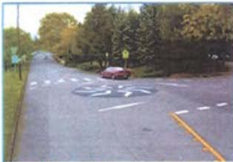
Photo 3. Potential improvement: Low-profile traffic circle.
